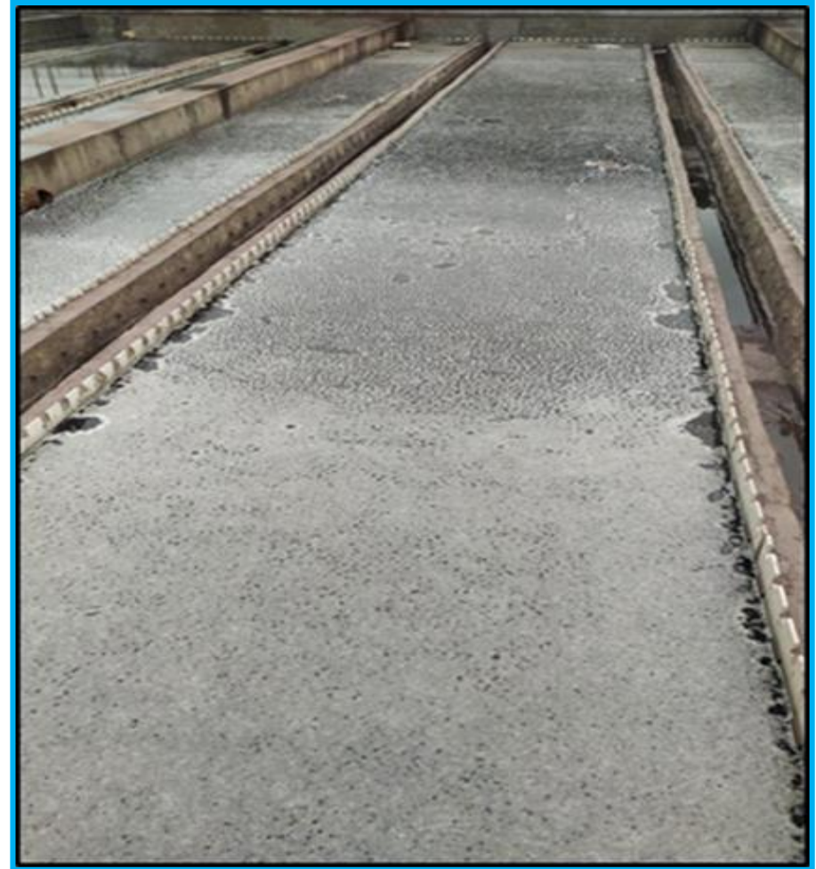
Pictorial view of Aerobic and anoxic treatment of BOD Plant Coke oven -2
