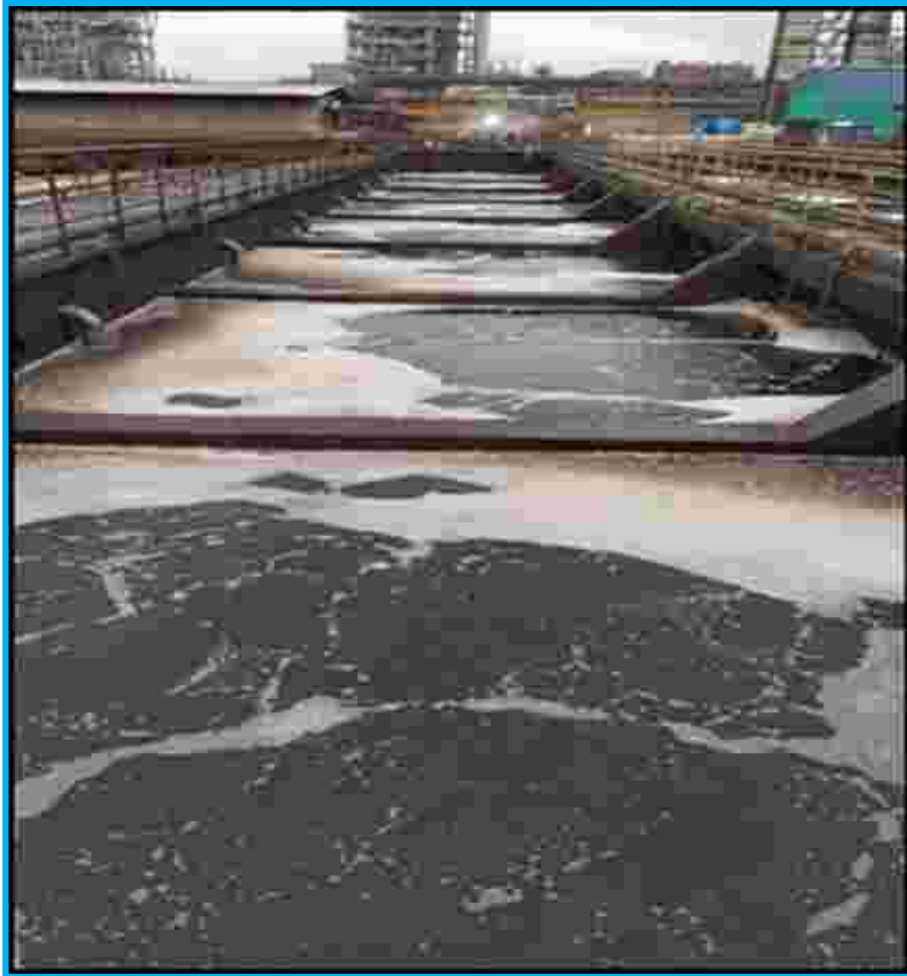
Pictorial view of Aerobic and anoxic treatment of BOD Plant Coke oven -2
